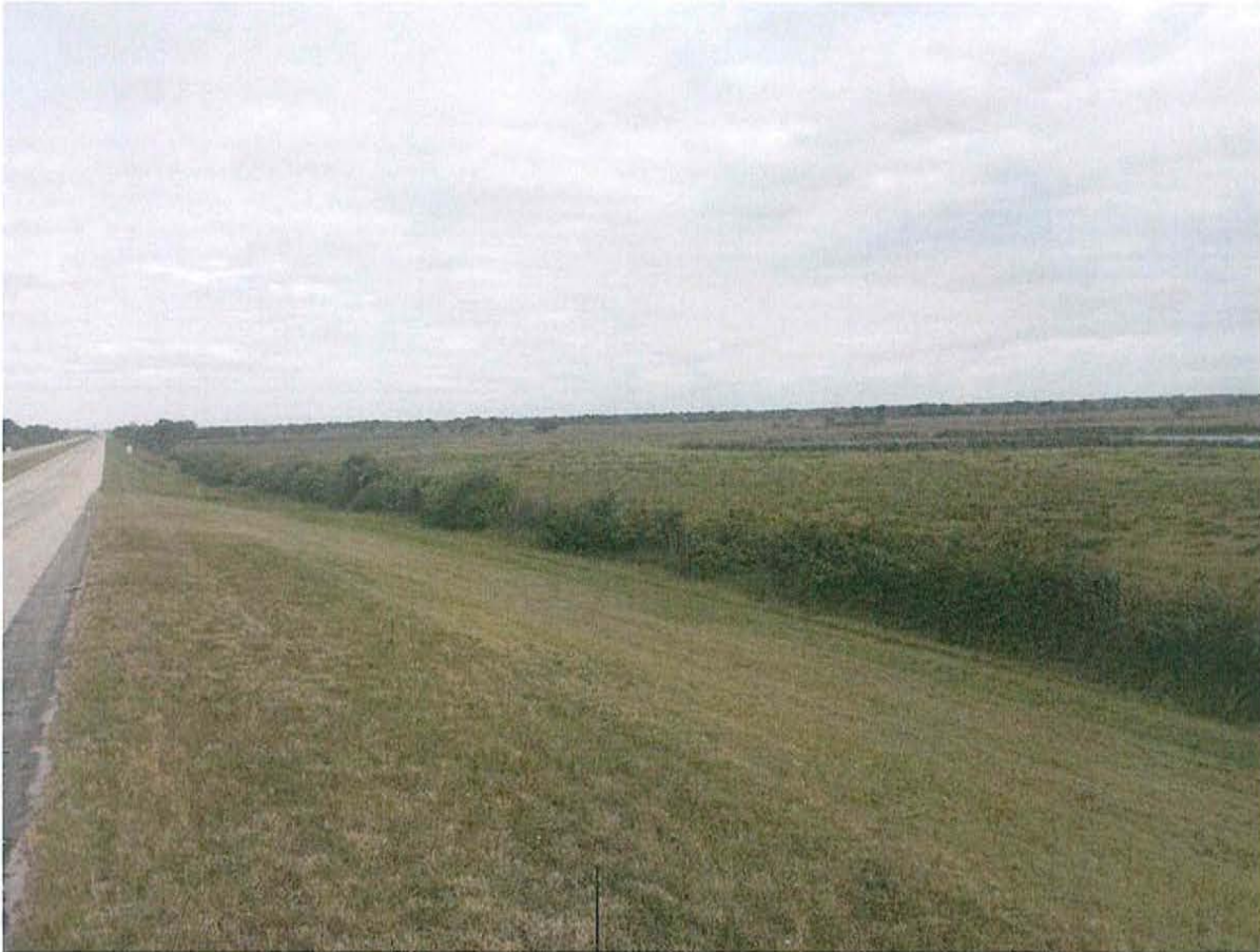
Northerly View along East Side of Highway 681; Subject at Right
